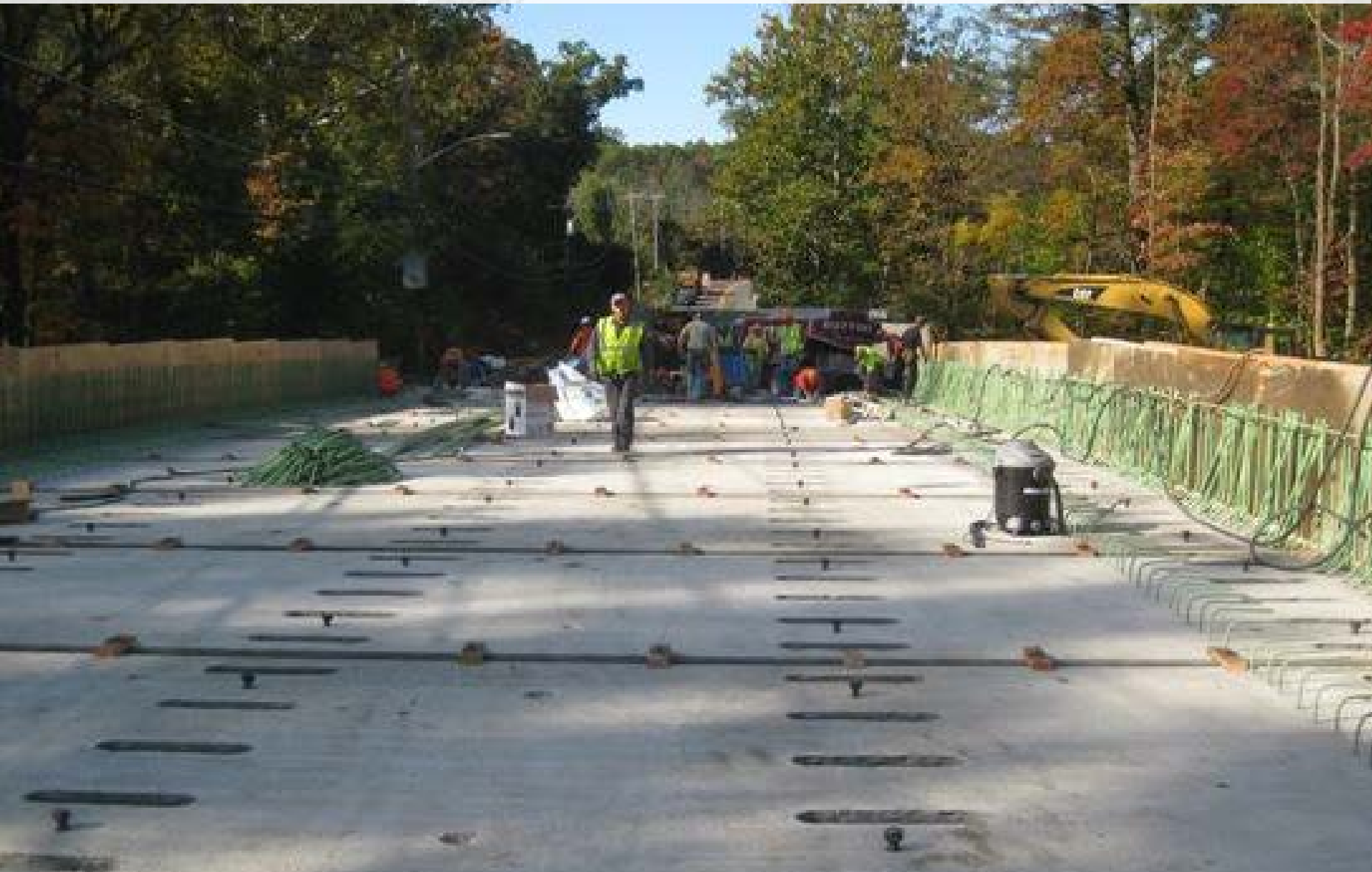
Example Construction- Bridges # 76 and 77 N&S
